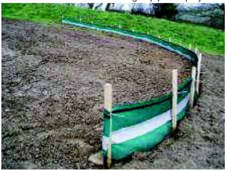
Hy-Tex Terrastop silt fence in use on National Grid's Felindre to Brecon gas pipeline project
